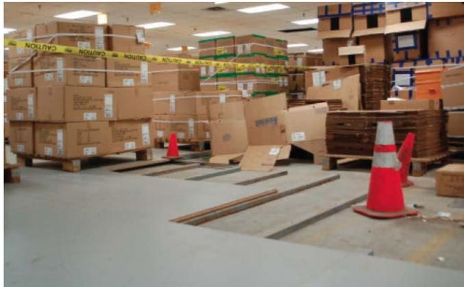
*Installation of ResinDek® and steel sleepers over damaged concrete*
