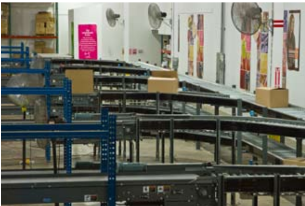
Two level MDR collection conveyors.
