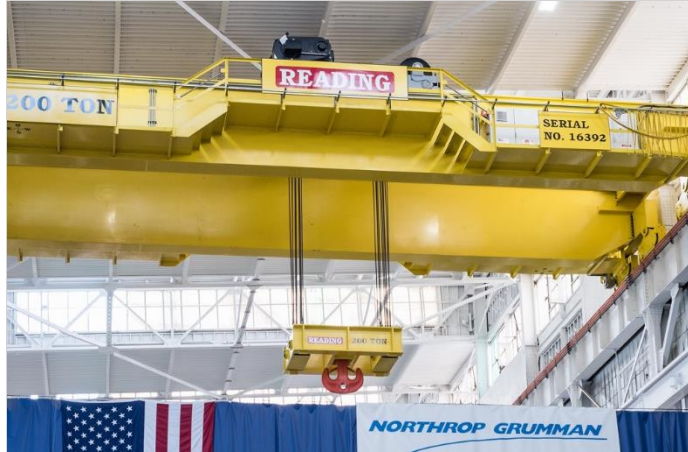
Reading Crane and Engineering Co. installed 200-ton crane with two 100-ton R&M Materials Handling, Inc. hoists at a Rhoads Industries facility.
