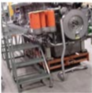
Assembly Floor Work Platforms
