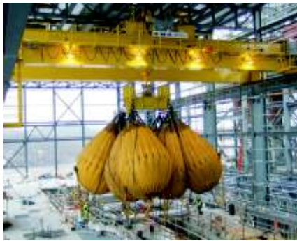
Overhead Bridge Cranes
