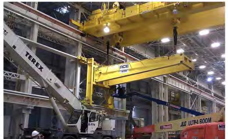
Custom engineered wall walking jib crane.
