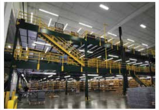
Custom mezzanine includes underground footplates and fewer columns to reduce obstructions.
