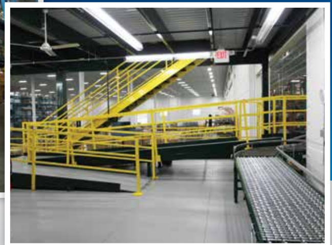
Custom catwalk and ramp designed to connect new mezzanine to existing mezzanine in adjacent building.
