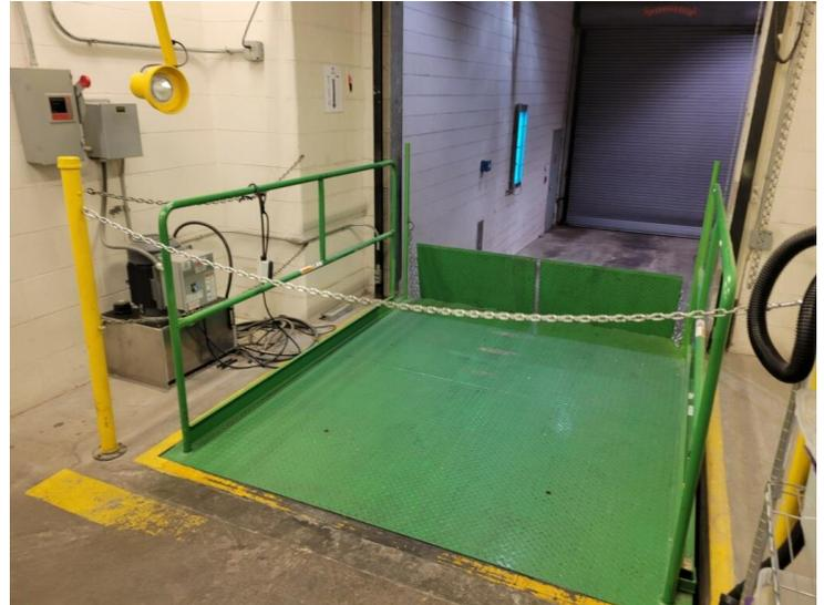
[Kelley KDL Series Hydraulic Dock Lifts](#) make product handling and loading operations more efficient in applications where space is restricted. Dock lifts are a cost-effective alternative to space-consuming concrete ramps and can accommodate a wide variety of truck sizes and styles from pickups to standard semi-trailers and more. Kelley KDL Series Hydraulic Dock Lifts can be pit or surface-mounted inside the building or in front of the loading dock for optimal versatility and feature:
