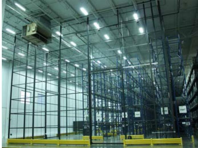
*The DEA cage for this application was designed to be flush to the floor of the facility and to reach the roof deck of the building; some 40 feet high.*
