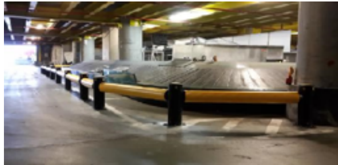
Barrier around baggage conveyor
