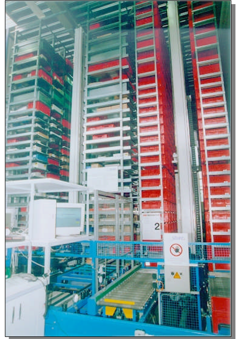
Mini-load with (2) viaspeed S/R machines with pin extractor load-handling devices.
