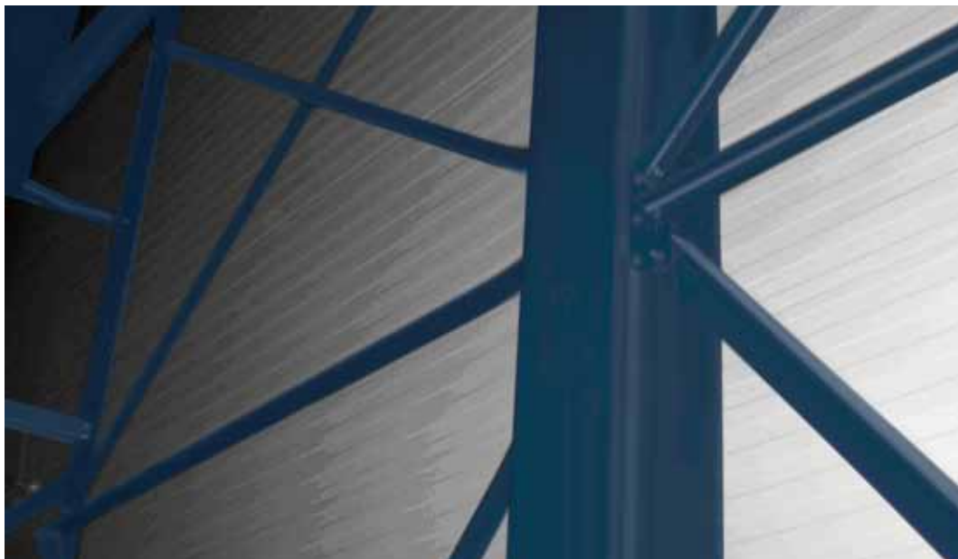
Special bracing system, horizontal and vertical, mounted upward from the floor throughout the entire frame. This dissipates the seismic energy generated by earthquakes.
