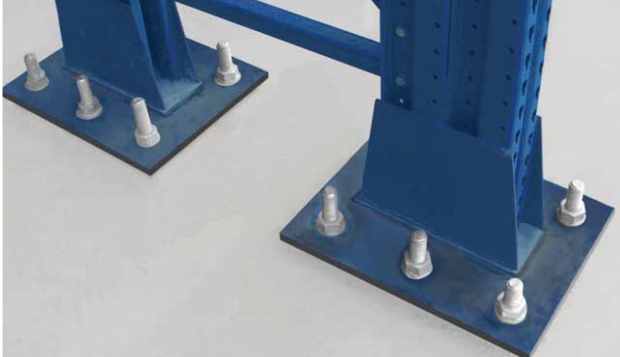
Anchor plates of larger dimensions and width provide greater resistance to traction.
