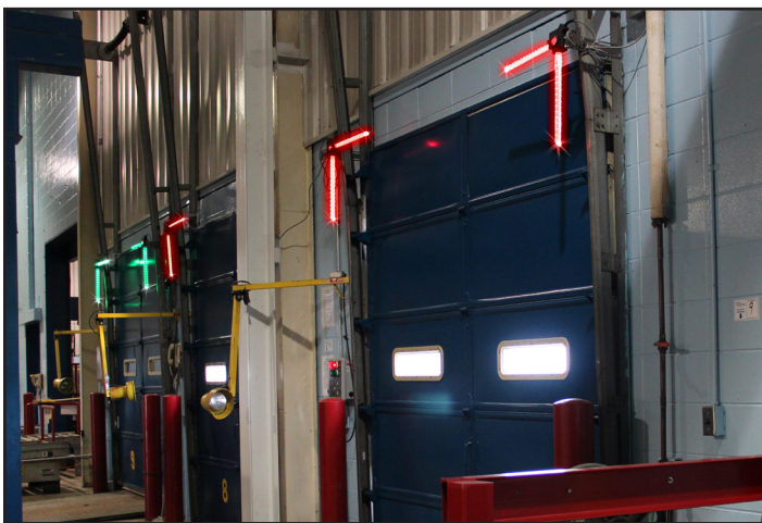
Corner-Vu lights (like those shown here) clearly indicate whether it is safe for a forklift operator to enter a trailer.
