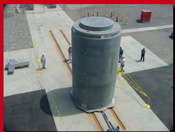
Cask is Clear of Containment Building Awaiting Pickup by Crawler
