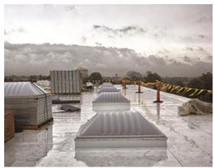
Prismatic lenses for skylights disperse natural sunlight into a facility more effectively. Combined with photocell sensors on high efficiency lights, such "daylighting" technology can cut lighting costs dramatically.
