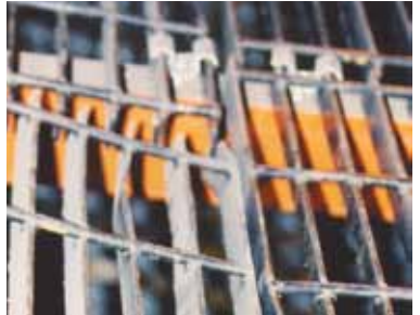
Deformed and damaged bar grate & plank grating
