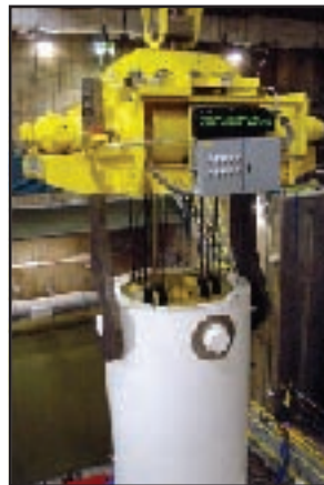
Canister Hoist Lowering
