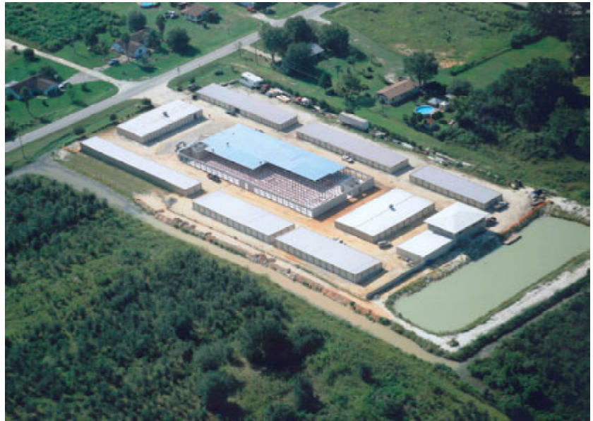
Aerial view of site during expansion to add a second level at AAA American Storage.
