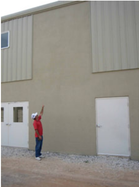
The ArmorCar VRC was installed through the roof and then used to move building materials up for final construction of the second level.
