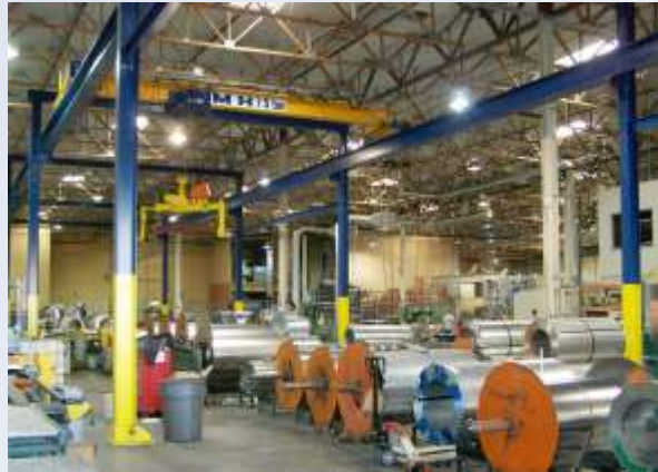
A 7.5 ton NOMAD system at a western manufacturer of ducting.
