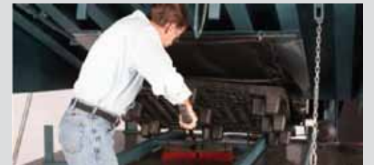
Easy clean leveler frame permits effortless clean out of pit floor.
