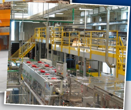
Mezzanine supports conveyor system and bottle line.
